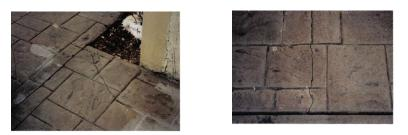
"Stamping" concrete is a common way of trying to achieve the attractive patterns associated with actual paving stone material. The stamping is done after the concrete has been poured and before it begins to harden. Stamped concrete is usually tinted (colored) before it is poured. There are standard colors that can be added to the concrete as it goes into the truck.
